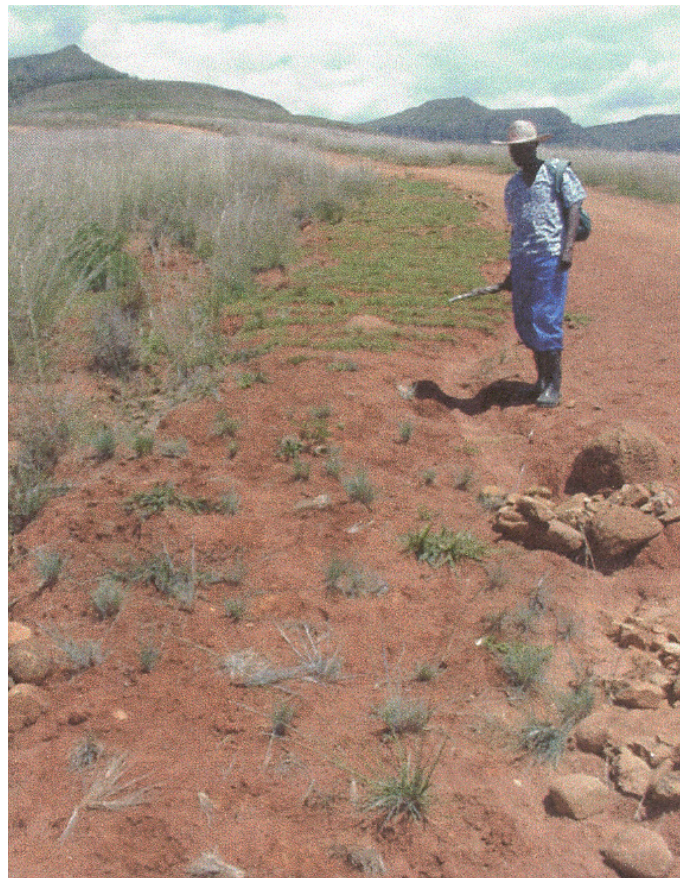
Plate 6. Indigenous grasses (lower slope) planted below Kikuyu (upper slope).
