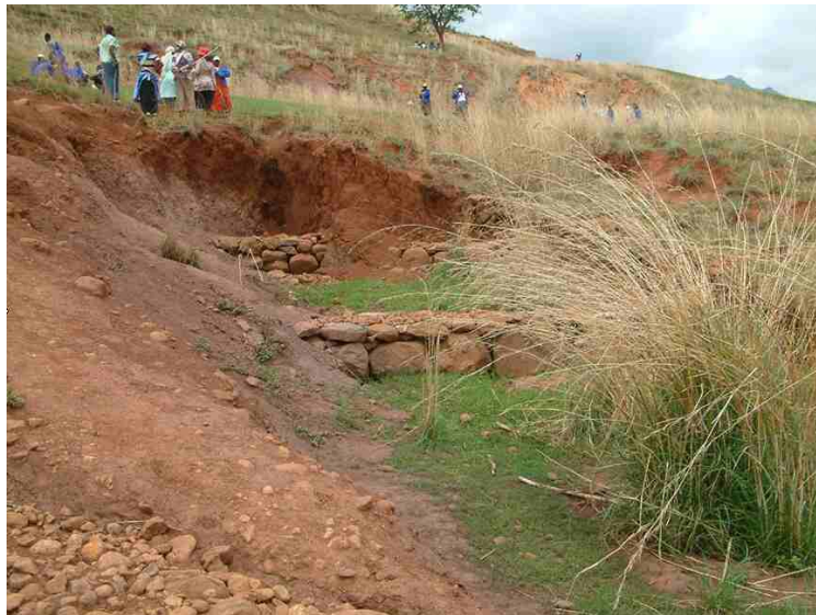
Plate 4. Stone lines across an eroded slope.
